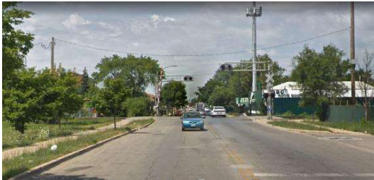
Existing condition on 71 st Street near Bell Avenue, facing west
